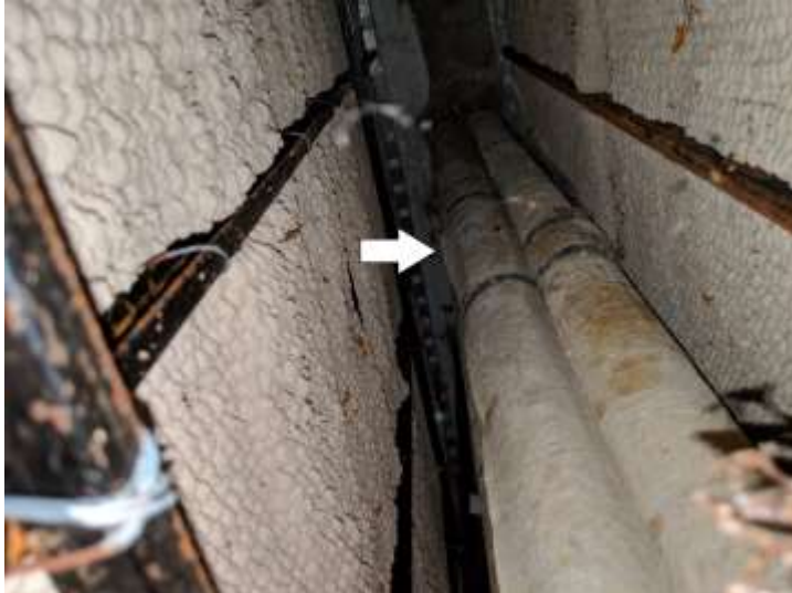
ACM Pipe insulation
